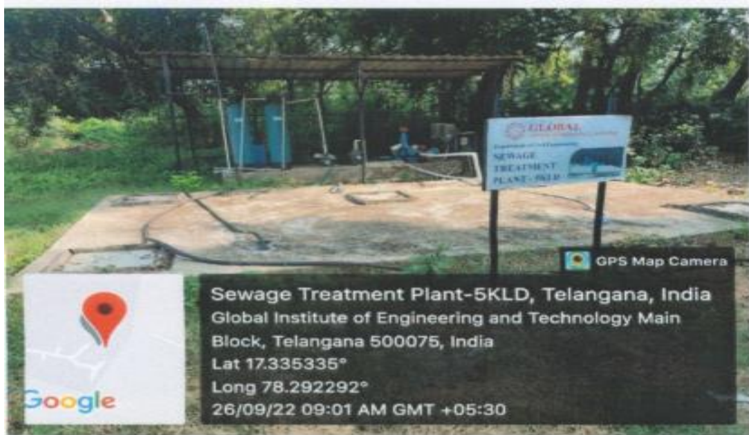
Sewage Treatment Plant in GIET Campus
