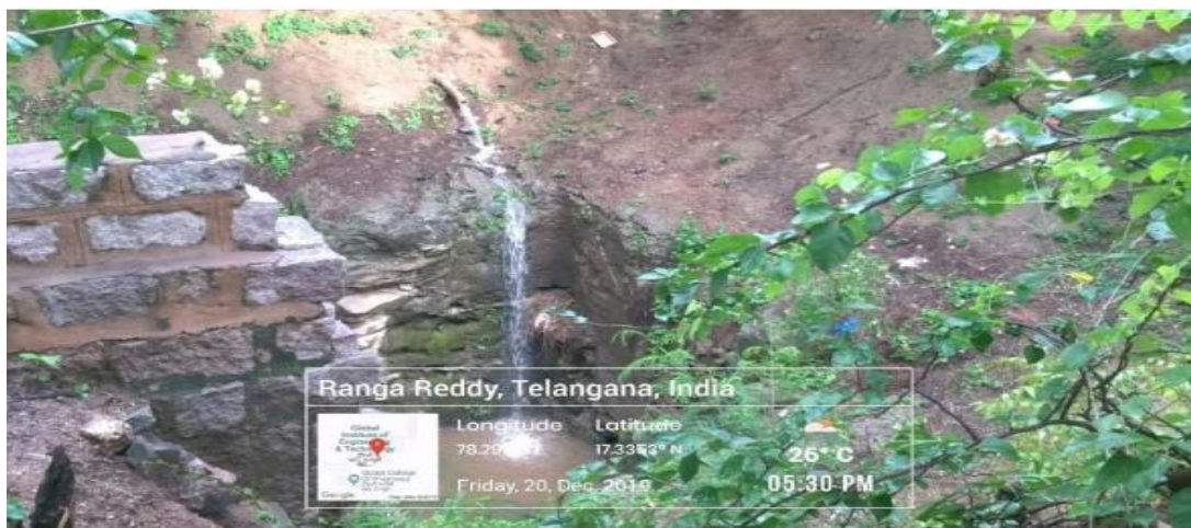
Rain water harvesting Pit
